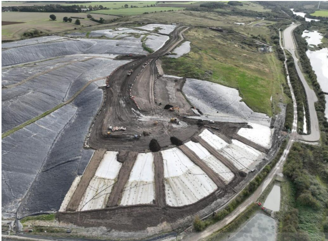
Permanent LLDPE Capping – Phase 13
