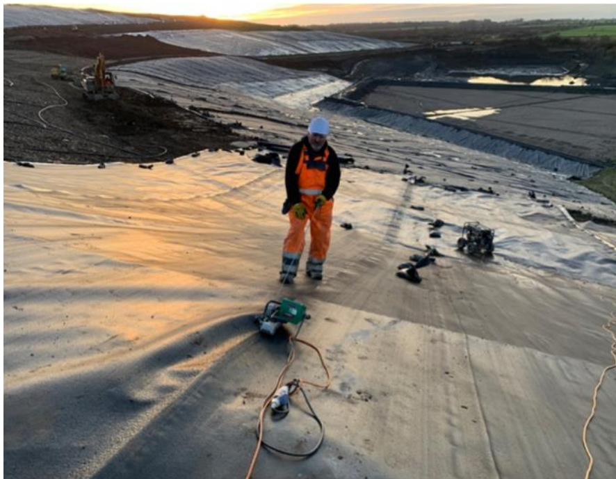
Phase 12 – LLDPE Capping & Pinning Location.
