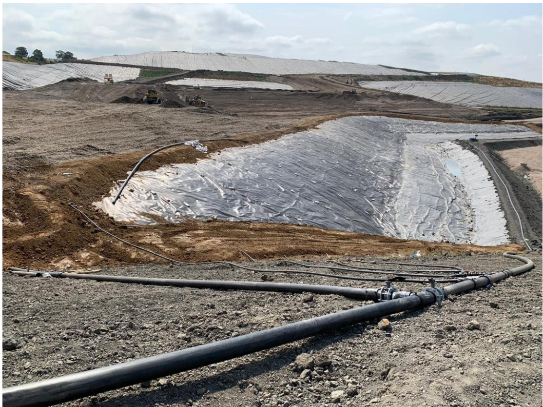
Recent capping works completed on phase 12
