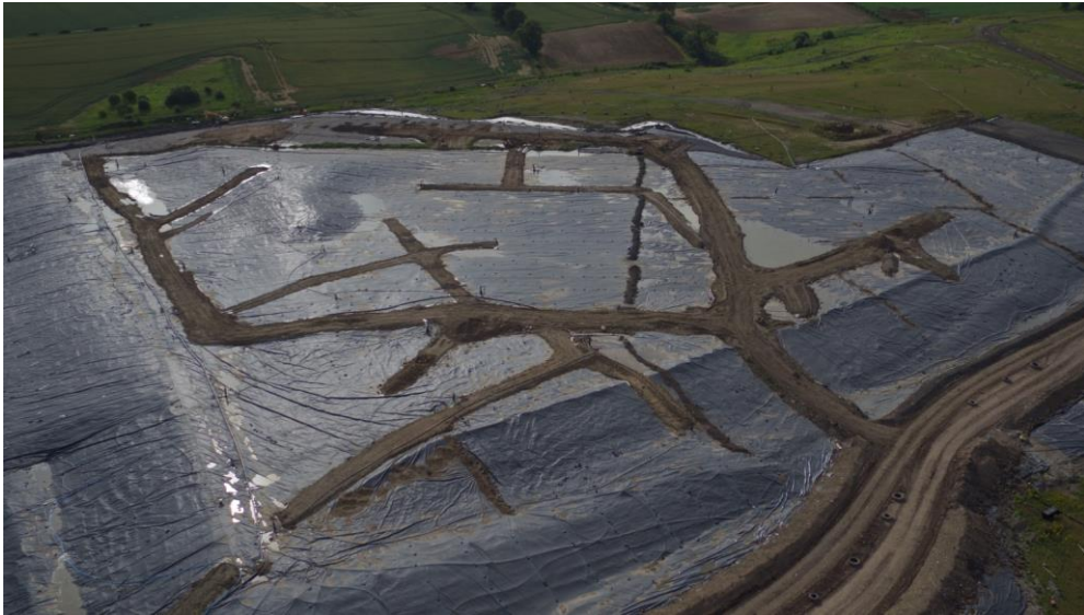
LLDPE Plastic Capping and soil spine roads.
