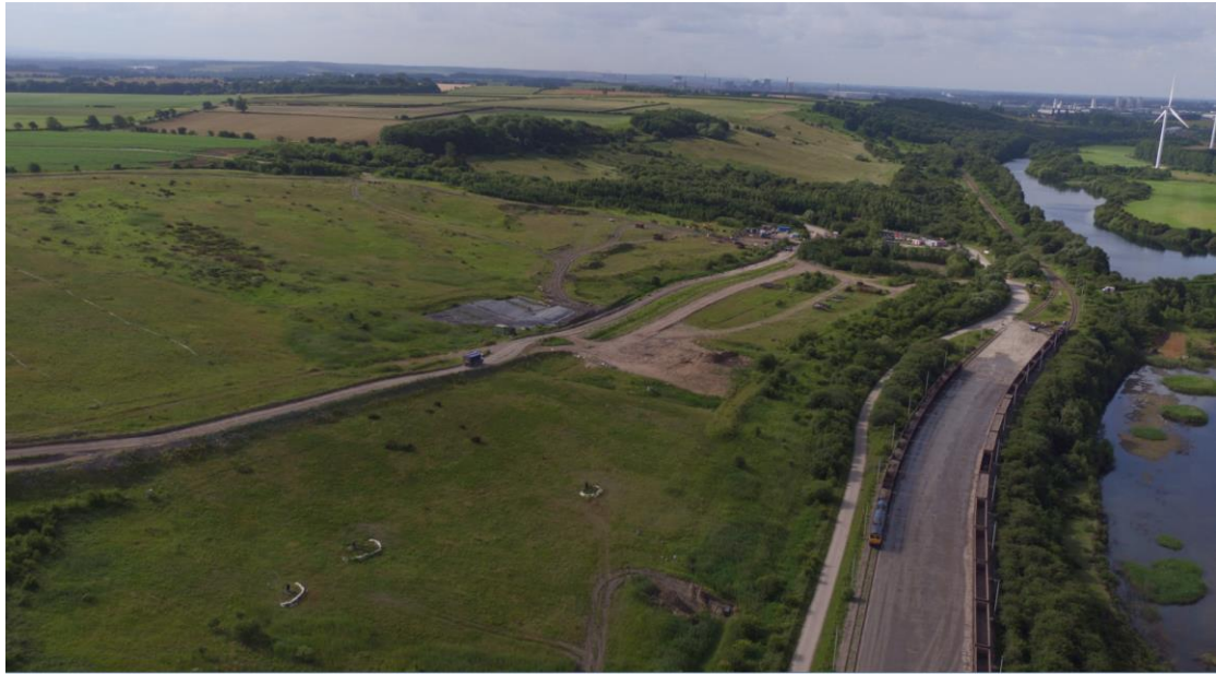
Rail Transfer Facility and restored area
