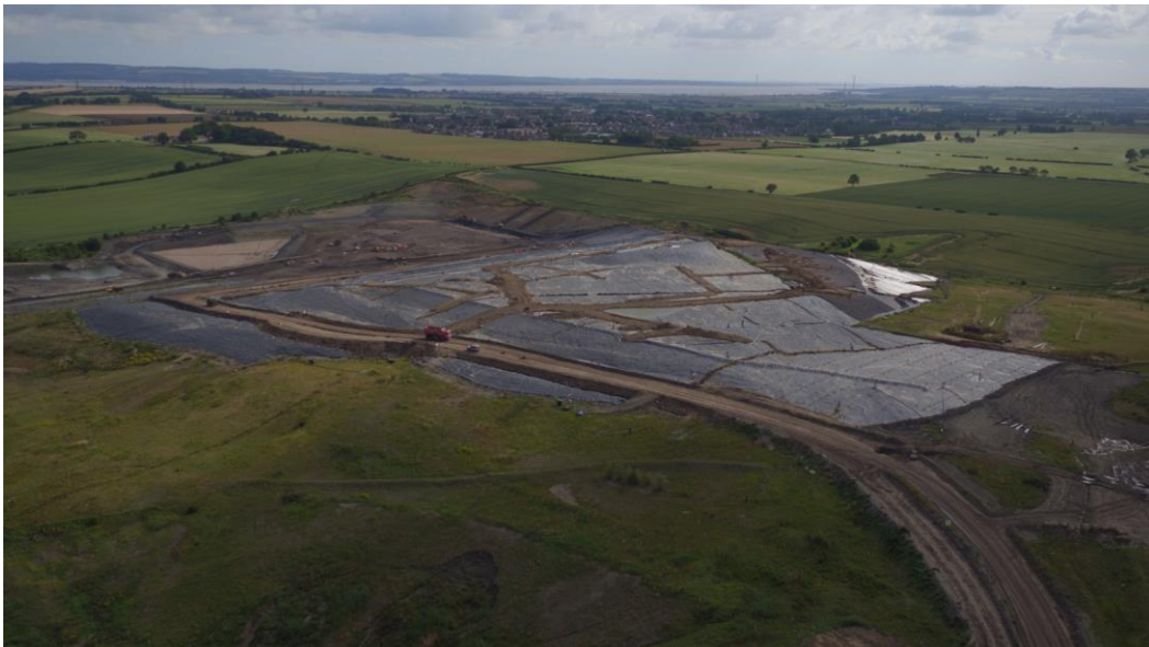
LLDPE Plastic Capping and restored areas
