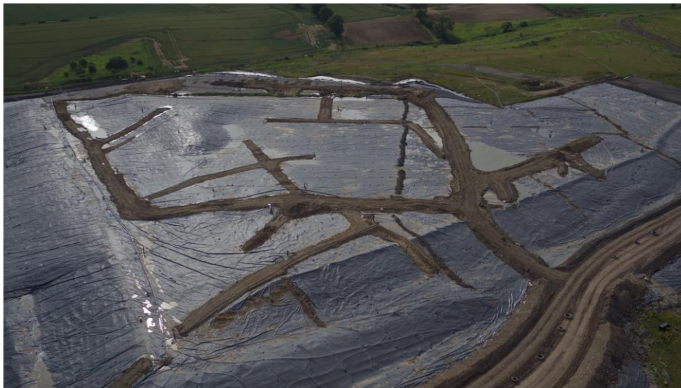
2019/2020 – LLDPE Plastic Capping and soil spine roads.
